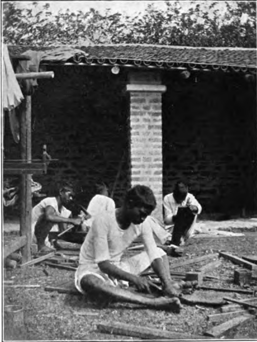
CARPENTERS AT WORK (p. 134)
